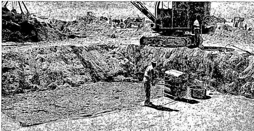
Figure A.9 Compacting backfill with gasoline-driven vibrating roller.
